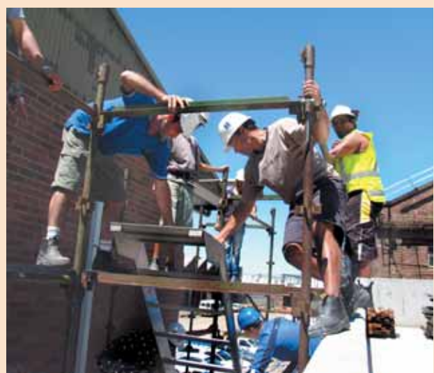
Students from the Course working on scaffolding.
